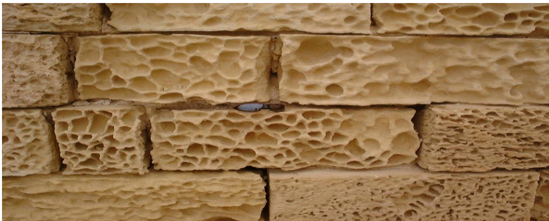
Fig No.Salt Weathering in Gozo
